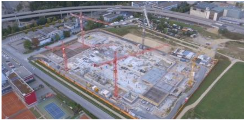
Innovation and production center, Biel, Switzerland
