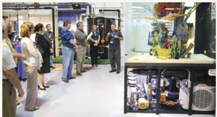
Guests at the opening of the new CoC in Irvine admire the saltwater aquarium with GF pipes.
